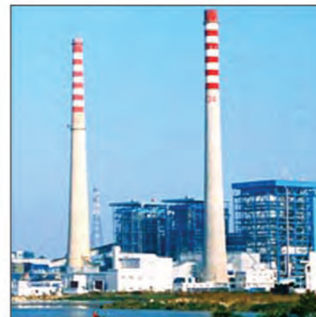
汕头华能电厂 Shantou Huaneng Power Plant
